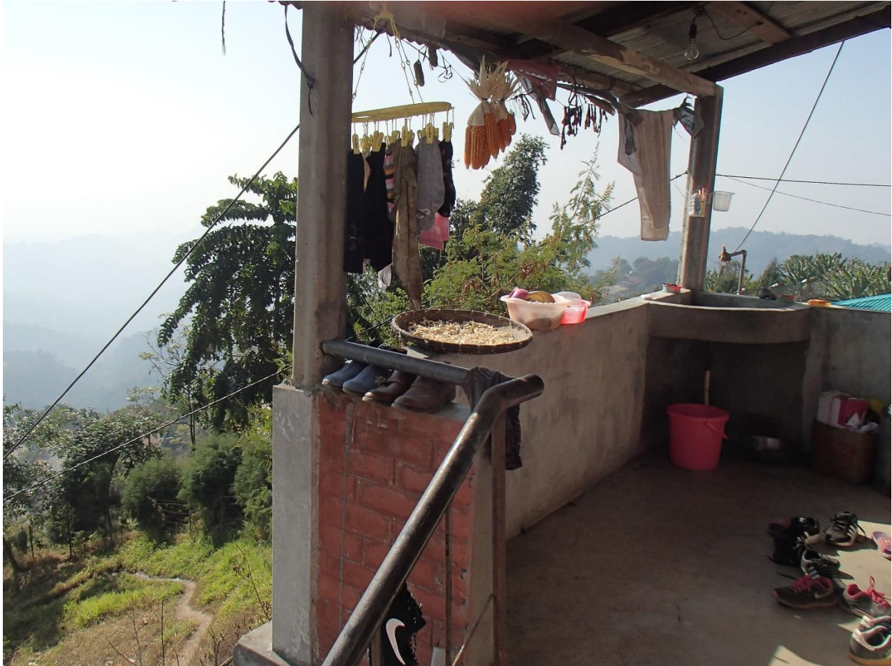
Figure 3. House landing. (J. Mitchell, Dewathang, Bhutan, 2017)
