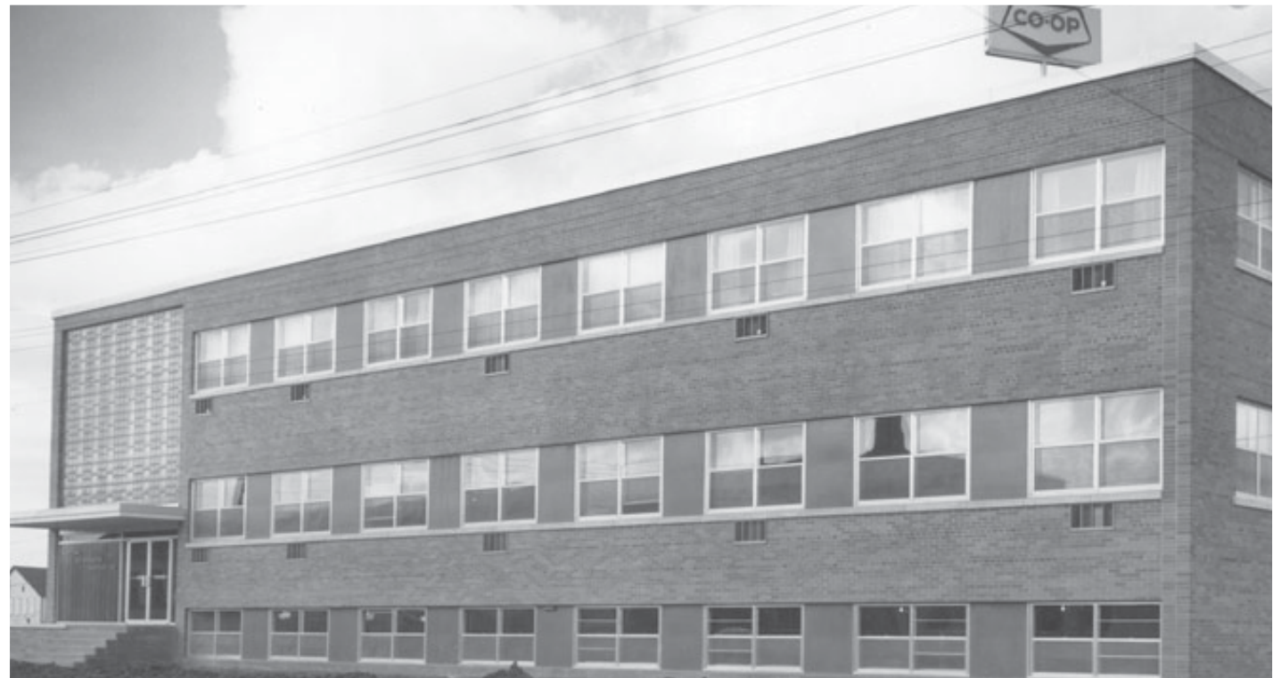
Moncton office building in 1969
